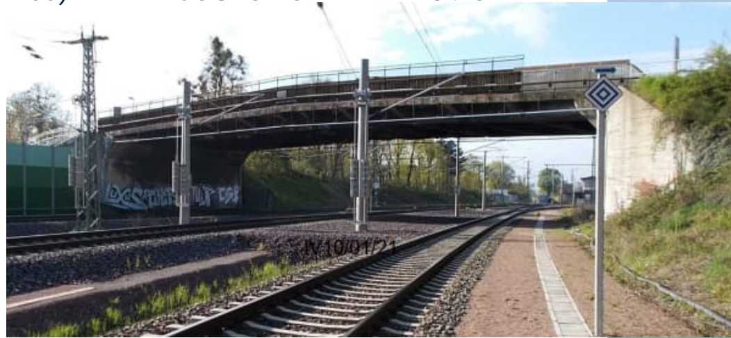
BRIDGE BEFORE REPLACEMENT
